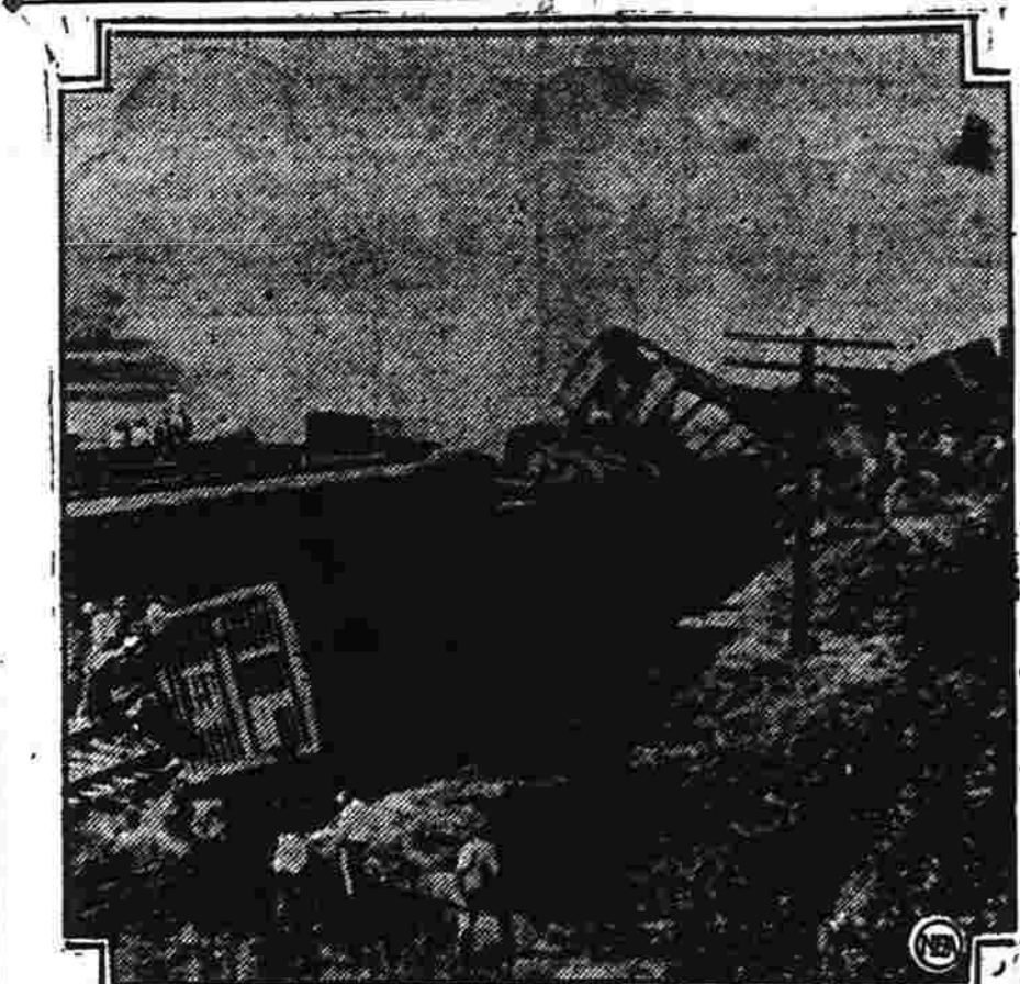
The pile-up of burning freight cars which followed the explosion of a locomotive of the Seaboard Air Line Railway near Petersburg, Va., is shown in this picture, taken immediately after the accident. Note the smoke and flames arising from the wreckage of the 50-car train as rescue workers arrived at the scene. Three men were badly scalded in the blast.
